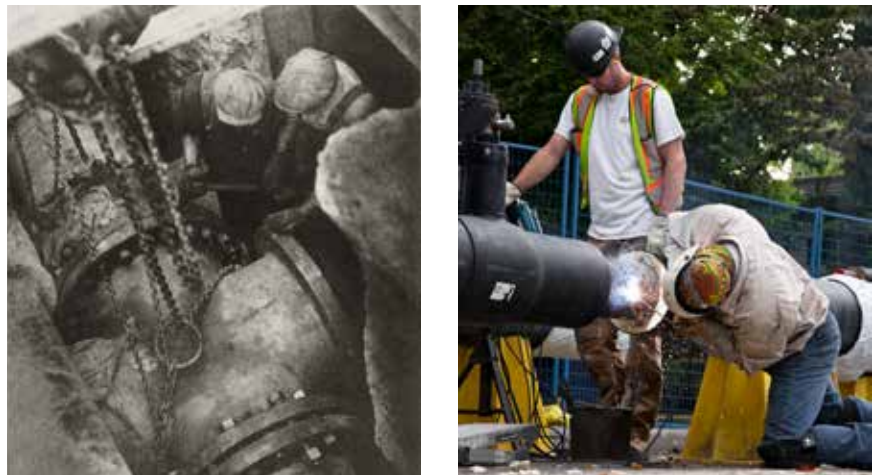
Installing a two-metre-diameter steam pipe for district heating in New York in the early 20th century (left). Welding a modern, pre-insulated district heating pipe in Vancouver (right).
