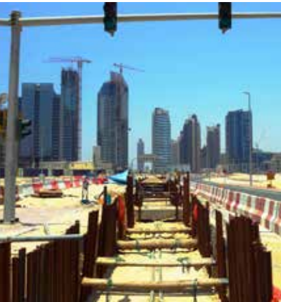
Laying district cooling pipes in Dubai, UAE.
